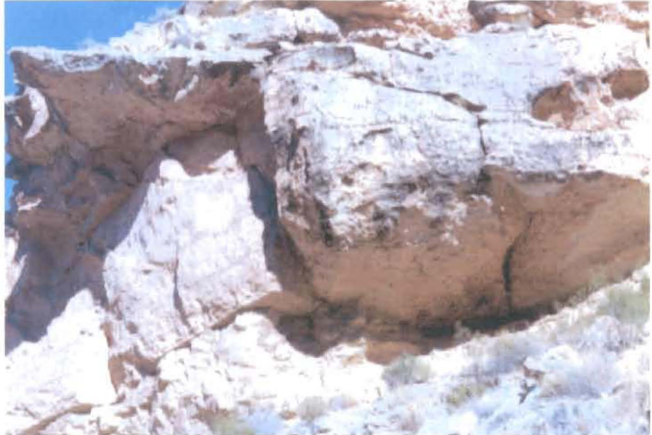
Photo 7: Mining was done here by digging out the entire ore layer until the overhang fell.
