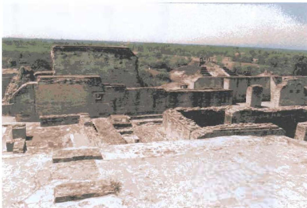
Figure 6: View across the Palace showing large window opening (at left and right) in East Wall (Photo: D. Eccott)
